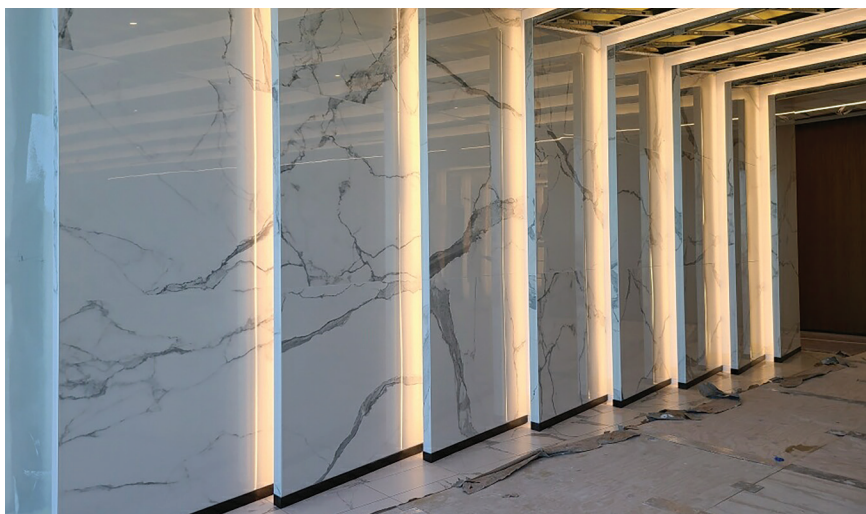
Reception feature wall: Rexi I Classico thin GPT panels.
